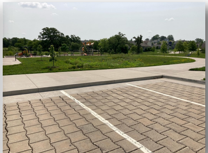
Image: Bioretention cell and permeable pavers in West Des Moines
