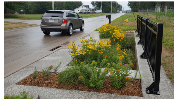
Permeable pavers (top) and bioretention cells (bottom) also soak in rainfall and manage stormwater where it falls instead of shedding polluted water.
