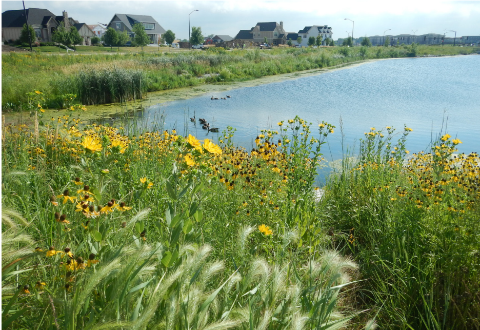
This pond is part of a series of natural treatment areas for stormwater. It was designed using the unified sizing criteria and it creates an open, park-like setting for residents to enjoy.
