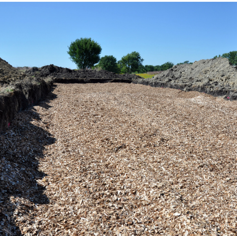
Woodchips serve as a carbon source for denitrification.
