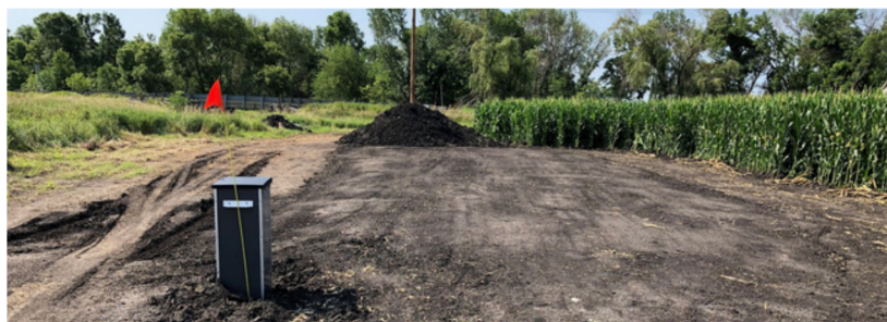
Woodchips serve as a carbon source for denitrification.
