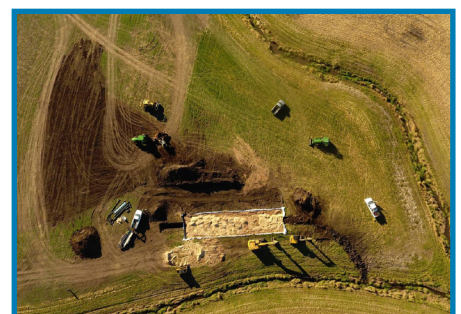
Bioreactor installation in Miller Creek Watershed - Black Hawk County photo courtesy of Kristi Heffelmeier
