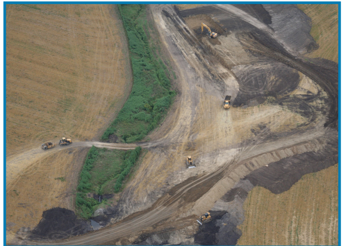
Construction of targeted wetland restoration in Wright County photo courtesy of Bruce Voigts
