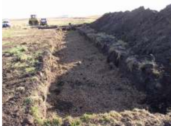
Installation of denitrifying bioreactor.
