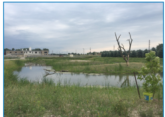
Stormwater wetland in Storm Lake
