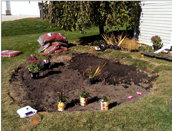
Step 3 Fill with amended soil
