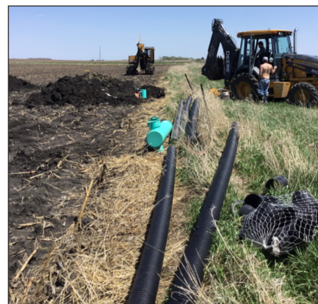
Saturated buffer installed in Buena Vista County
