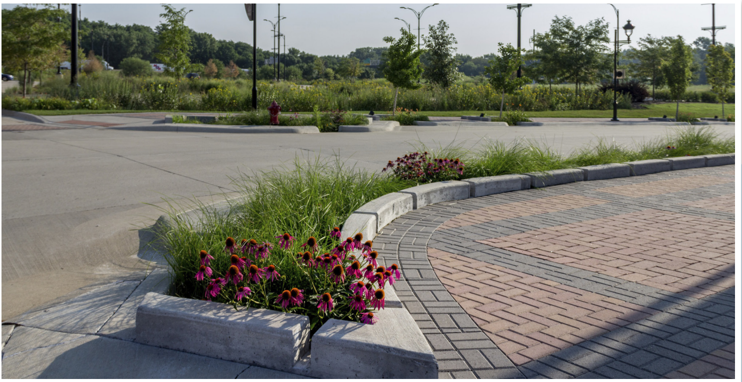
Coralville Bioretention Cells and Permeable Pavers
