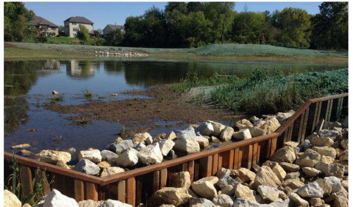
Stormwater wetland outlet near residential area in Easter Lake
