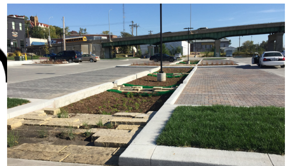
Permeable Pavers & Bioretention Cells Ottumwa, IA
