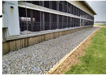
Infiltration Trench Dairy Robotics Center Calmar, IA
