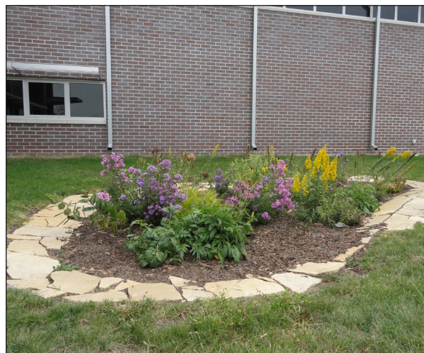
A rain garden at a new fire station in Coralville infiltrates roof runoff. Another bioretention cell manages parking lot runoff at this site.
