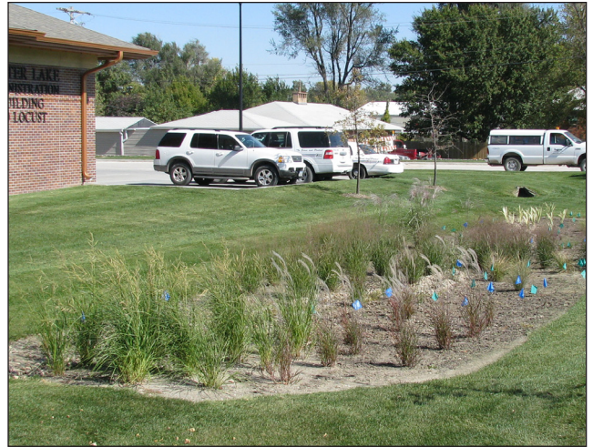
Carter Lake City Hall added a bioretention cell to manage stormwater. The Carter Lake Watershed project was recognized by EPA for its success.
