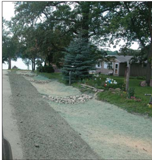
This is one of the many road ditches that were converted to bioswales that convey water to biocells in East Okoboji Beach – a rural subdivision on the east side of East Okoboji Lake.
