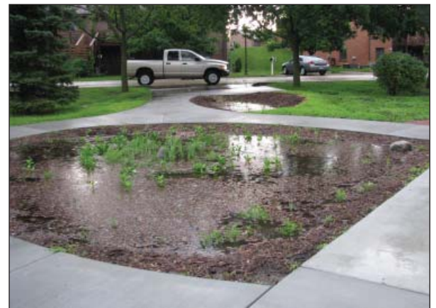
Water is temporarily impounded in this rain garden located at an assisted living facility in Council Bluffs.
