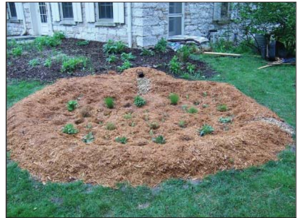
A rain garden installed at the University of Iowa by UI Engineers for a Sustainable World, with assistance from Johnson Soil and Water Conservation District.
