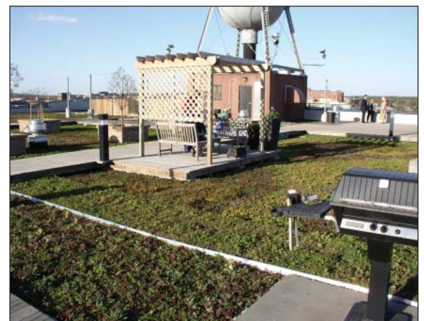
This green roof on Water Tower Place - a warehouse renovated to offices and condos - provides charming green space for residents, while reducing roof runoff.
